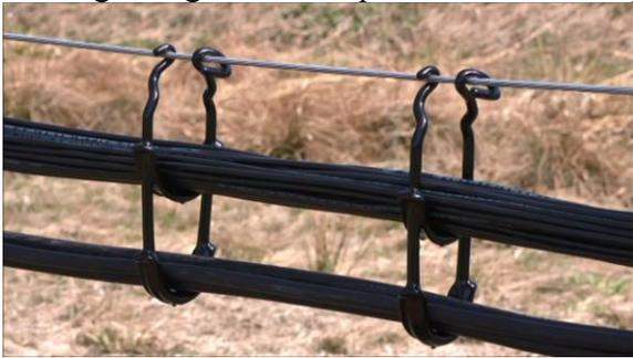
Figure 3: Single Cable Ring with Two Saddles
