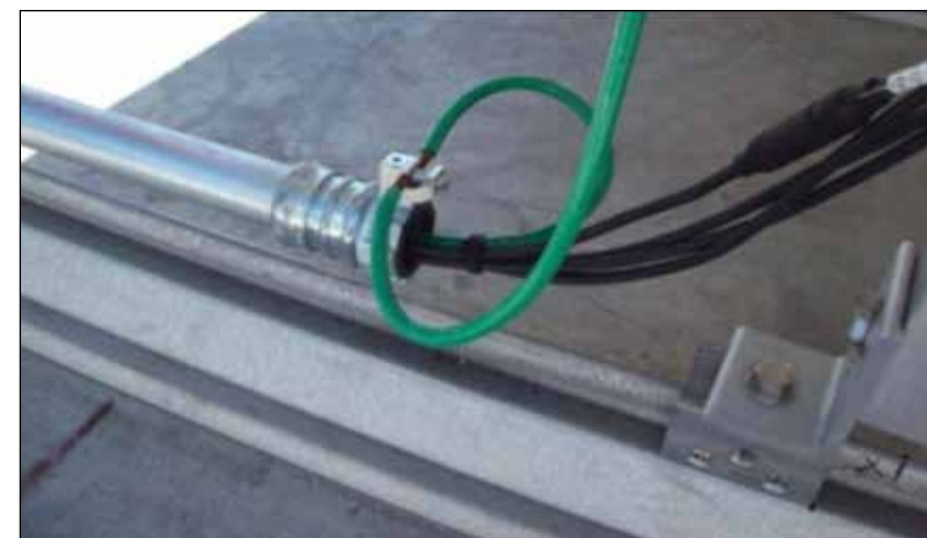
Figure 4. Exposed USE-2 cable protected and supported using EMT.
