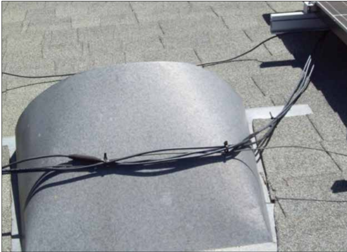
Figure 5. Insufficiently protected and supported USE-2 cable on a roof exposed to physical damage
