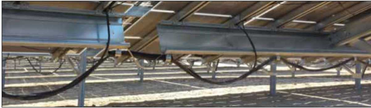
Figure 9. 10 AWG USE-2 cable with 4.5' distance between supports
