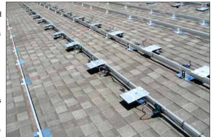
Figure 1. Large micro-inverter cable system prior to PV module mounting. Photo courtesy of Enphase Energy.
