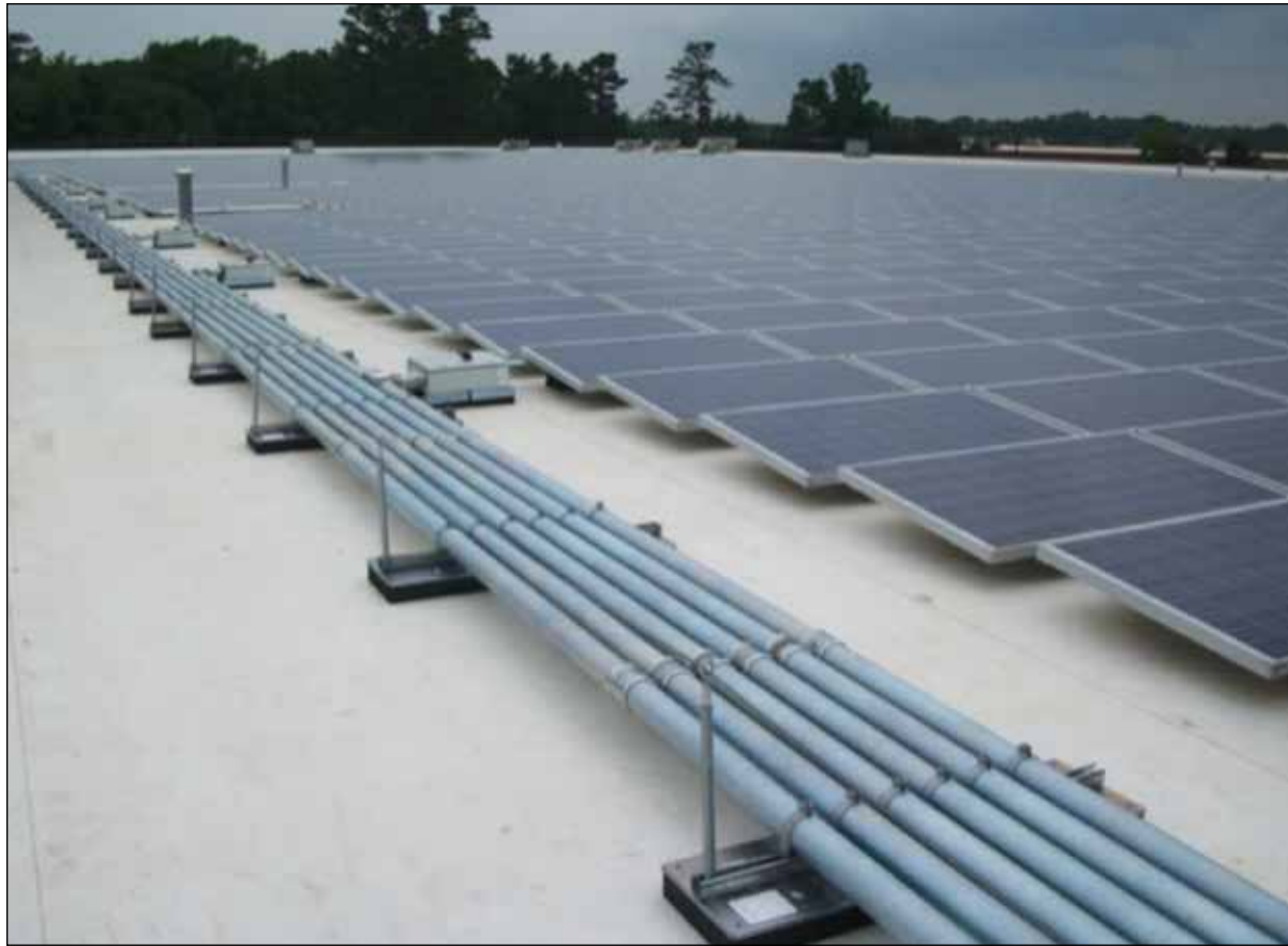
Figure 2. PV output circuits in EMT on commercial roof
