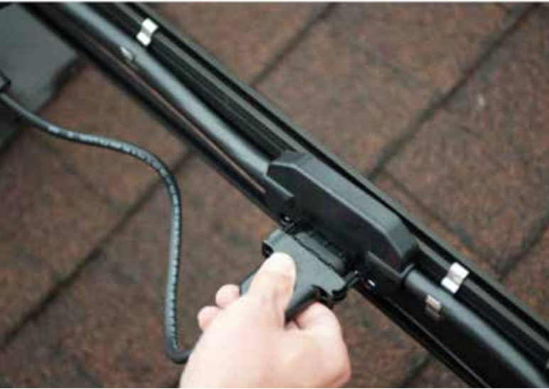
Figure 12. Factor cable assembly with proper support. Photo courtesy of Enphase Energy.
