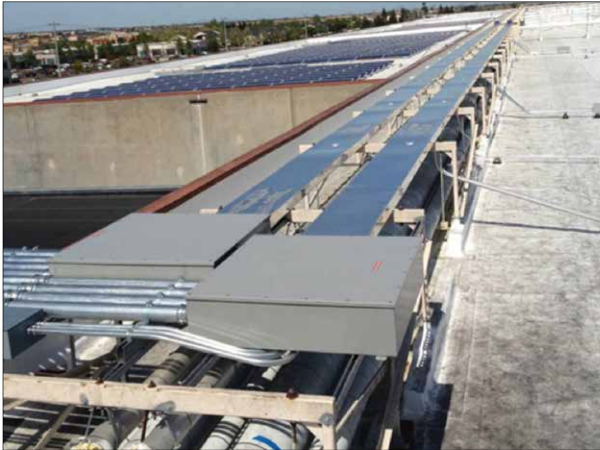
Figure 6. PV output circuits in covered cable tray on commercial roof
