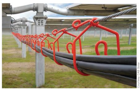
**Messenger-wire cable support** CAB Solar has developed more than 25 unique designs for cable rings and saddles that safely support large bundles of string wires, dc and ac feeders, data, grounding conductors or other cables.
