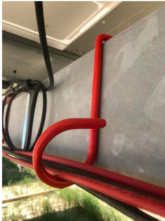
Figure 3: Torque Tube Hanger Supporting String Conductors
